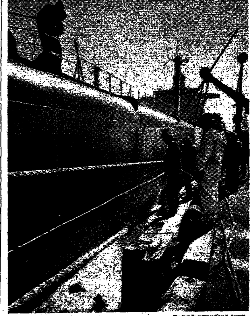
TRYING TO PLUG THE HOLE: Divers at dock in Perth Amboy, N.J., attempting to repair gash below water level in oil tanker, Richard C. Sauer, of Liberian registry. After hull was pierced yesterday, about 250,000 gallons of oil spilled into the Arthur Kill.
